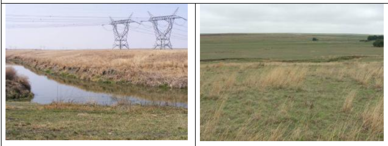
Waterval River showing existing power line crossings
